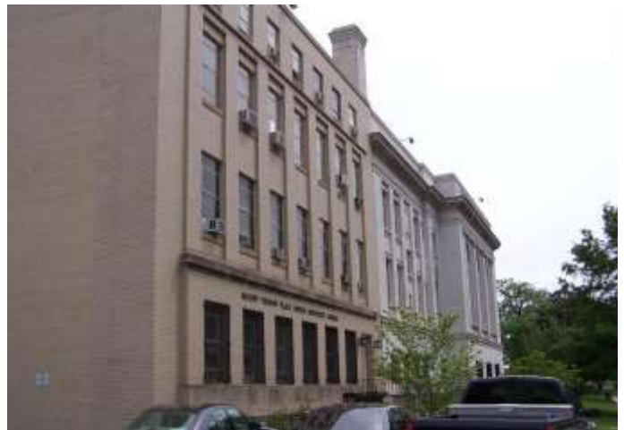
2005 View from K Street, NW
